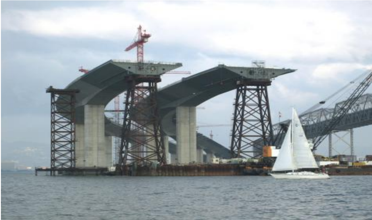
Second Niger Bridge project
