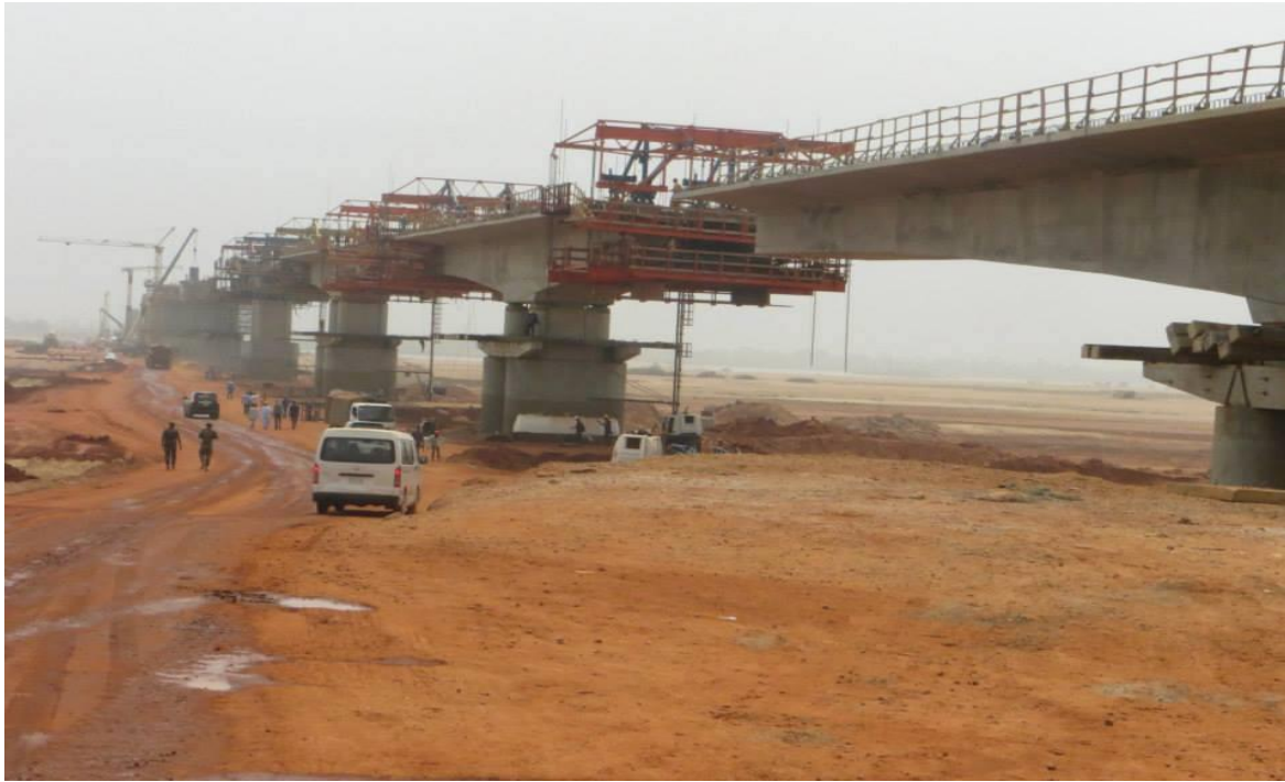
Second Niger Bridge project
