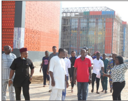
Facility tour of the construction site
